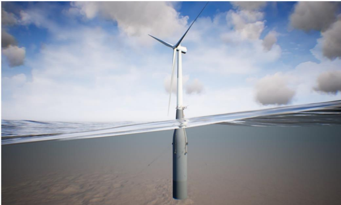
Figure 3-2: Hywind Tampen Concrete Foundation (Credit: Equinor)
