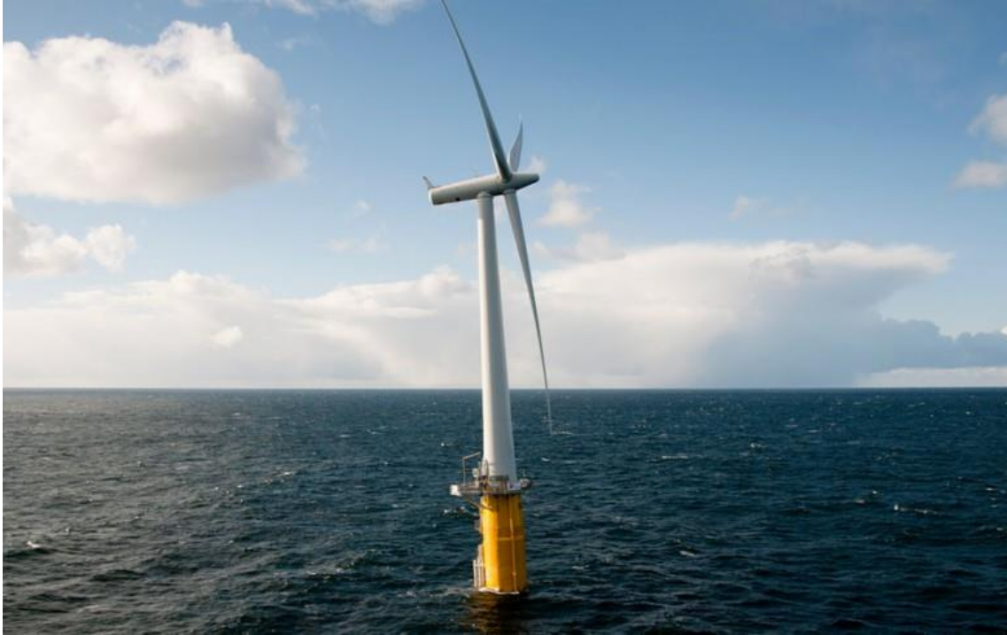
Figure 4-3: Hywind Demo Offshore Floating Wind Tower
