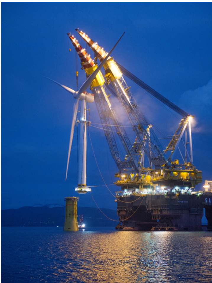
Figure 6-6: Hywind Scotland Pilot Park Installation (Credit: Equinor)
