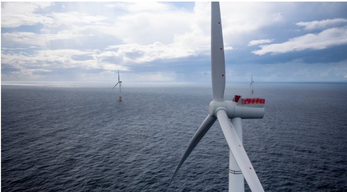
Figure 4-1: Hywind Scotland Floating Offshore Wind Farm (credit: Equinor)
