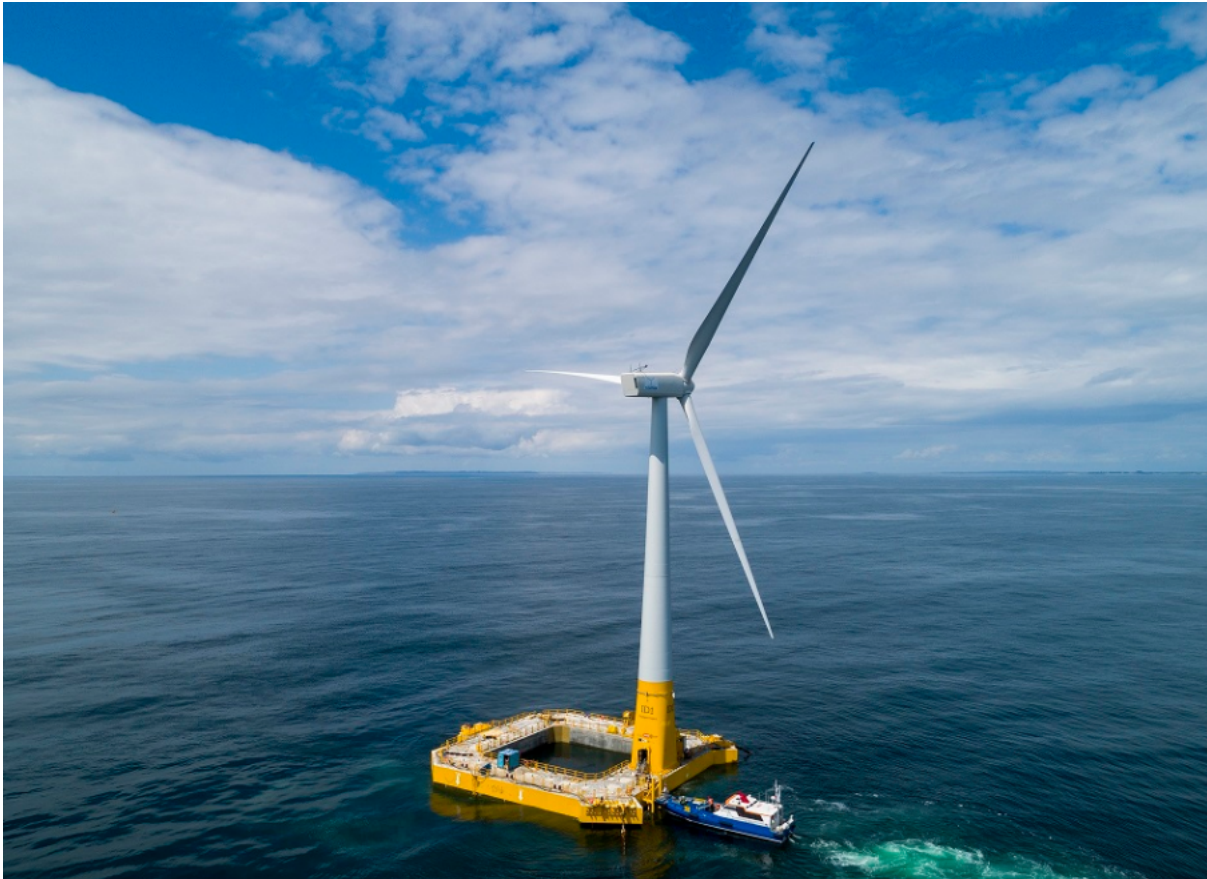
Figure 4-4: Floatgen Demonstrator Towing to Location (Credit: Ideol)
