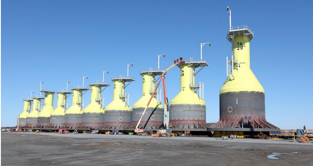
Figure 6-3: Gravity-based Foundation for Tahkoluoto Wind Farm (Credit: Offshorewind.biz)
