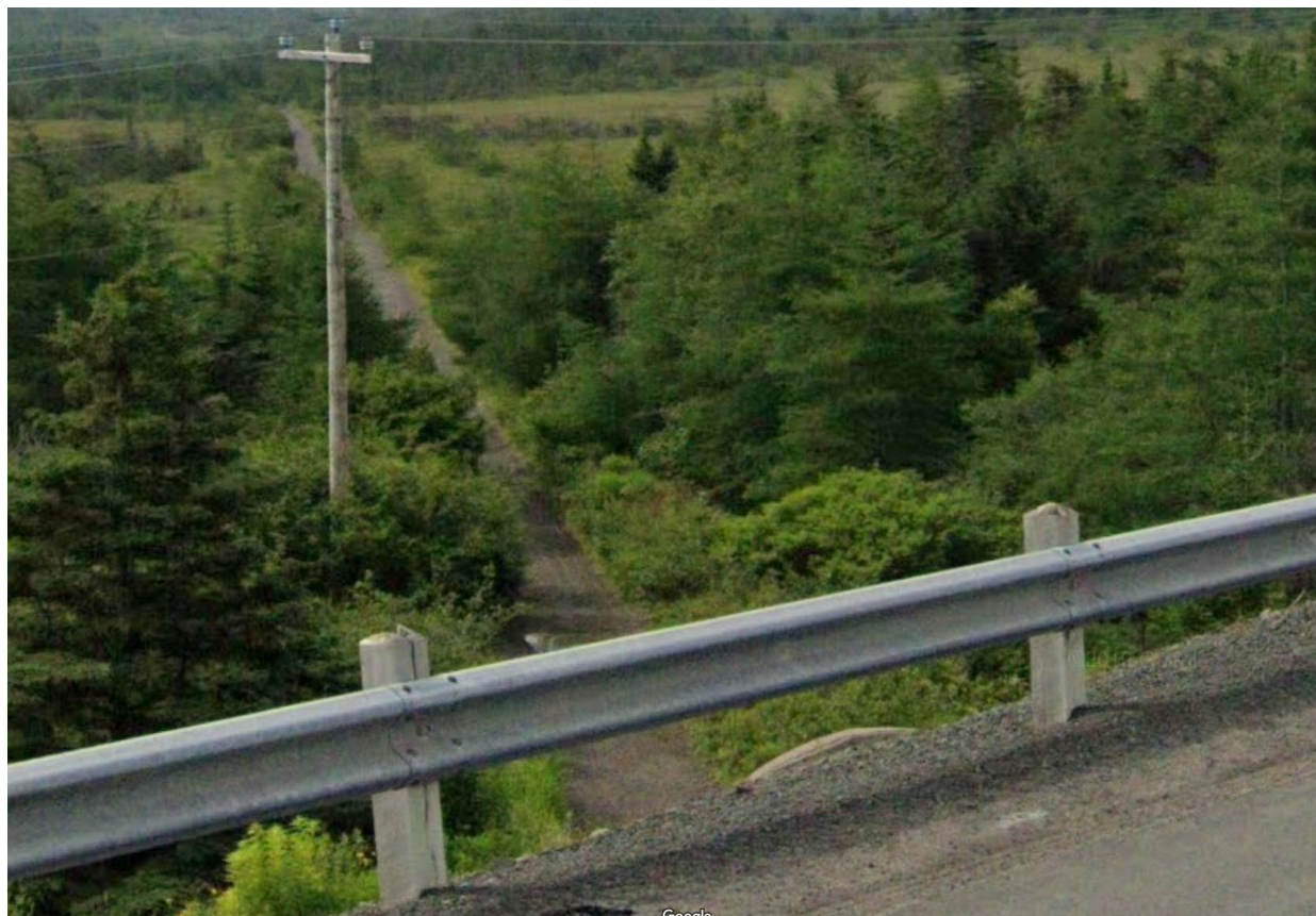
Figure 4. NL Trailway TCH underpass near Come by Chance refinery
