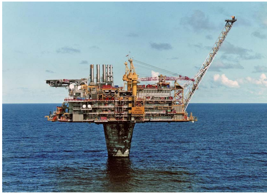
Figure 11-10 The Draugen platform ( www.norskipetroleum.no )
