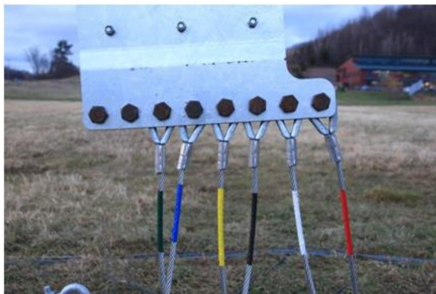
Picture 3-57: Correct lifter attachment to rocker plates (60 m tower)
