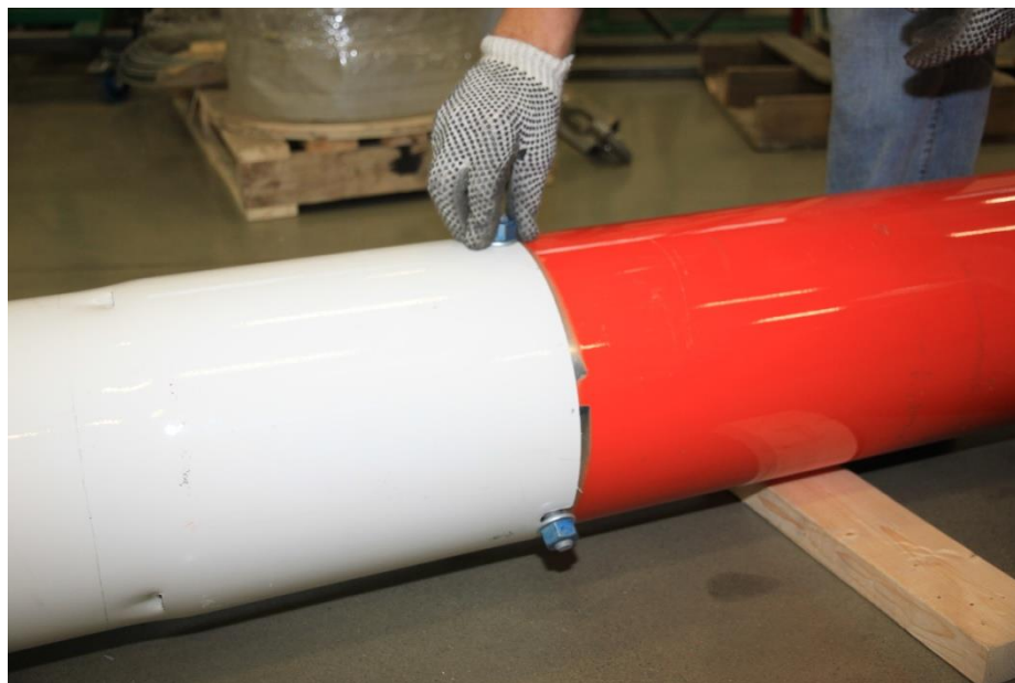
Picture 3-20: Nuts/bolts hand tightened
