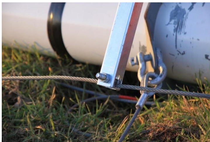
Picture 3-50: Threading the jumper strut cable
