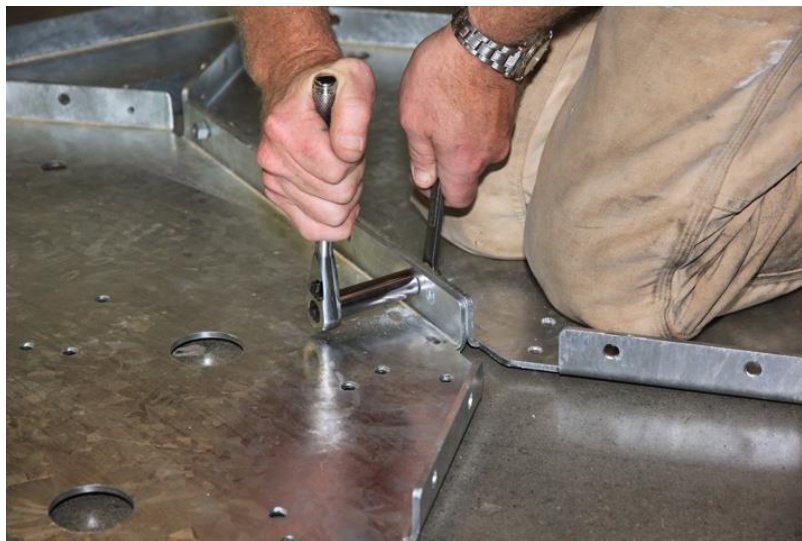
Picture 3-2: Baseplate Assembly
