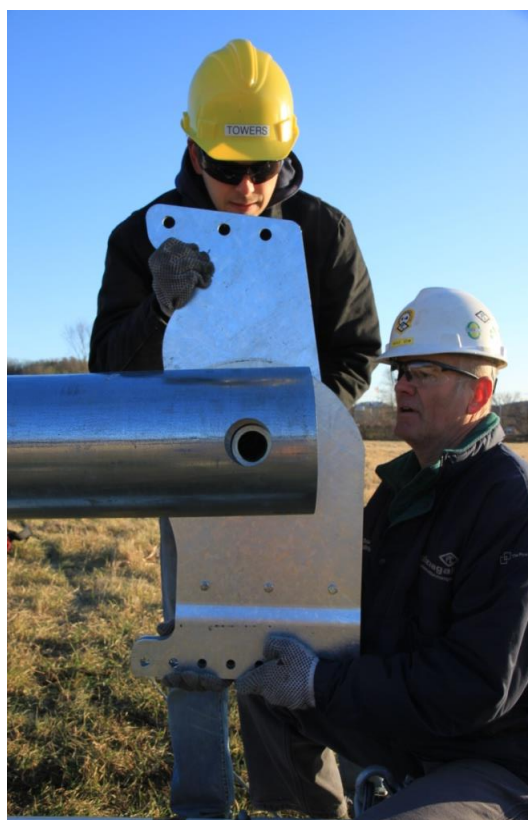
Picture 3-54: Ginpole rocker plate assembly
