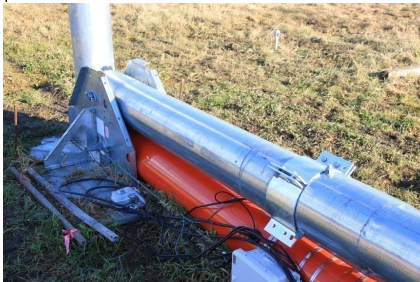
Picture 3-40: Ginpole jumper strut end-flanges
