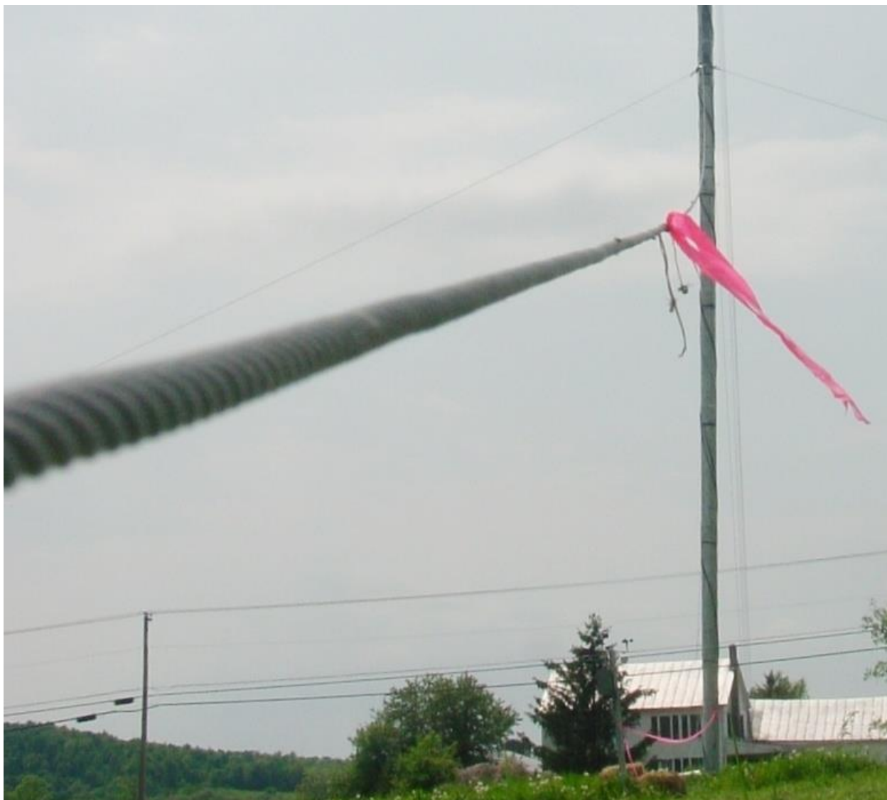
Picture 4-7: Level 1 guy, sag = 1-1/4 tube - just right
