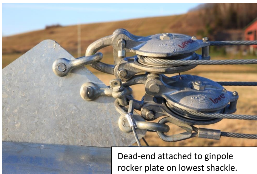
Picture 3-78: Affixing dead-end to ginpole rocker plate
