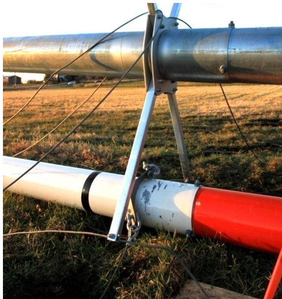
Picture 3-49: Threading the jumper strut cable
