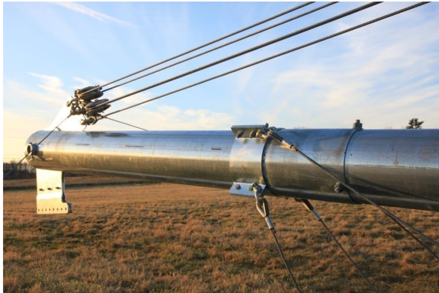
Picture 3-47: Jumper strut cable attachment
