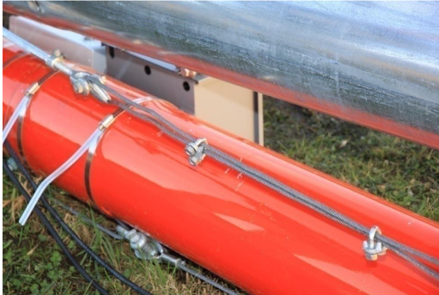
Picture 3-51: Attach jumper strut cable to turnbuckle
