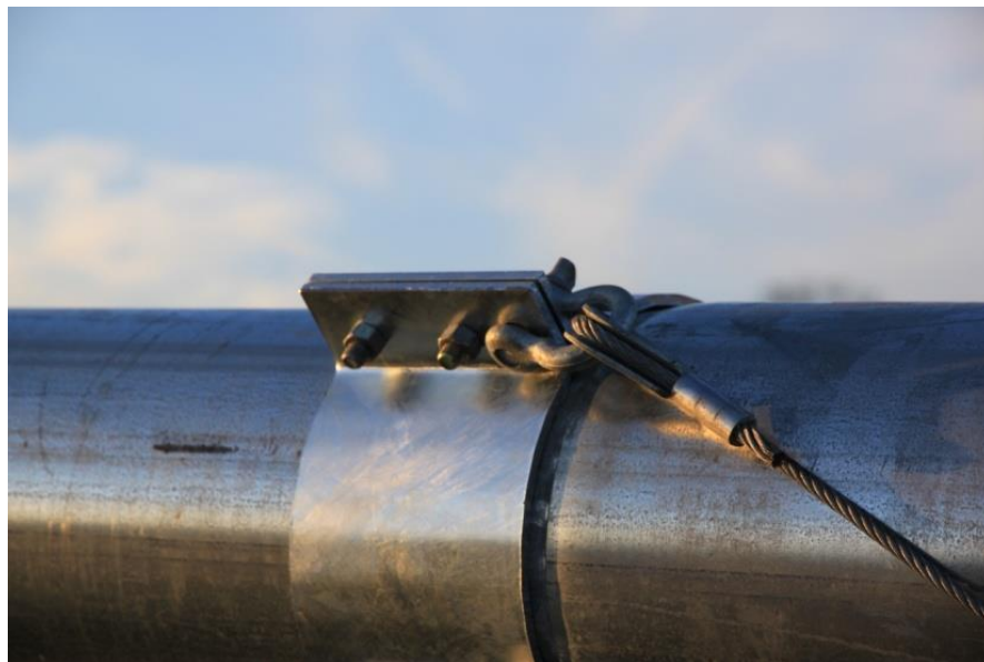
Picture 3-48: Jumper strut cable attachment detail
