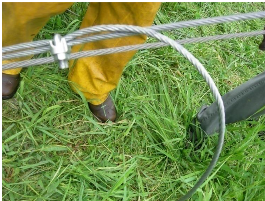
Picture 3-34: Wire rope clip guy wires together at anchor points
