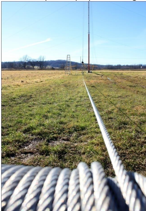
Picture 3-68: Correct winch cable fleet angle
