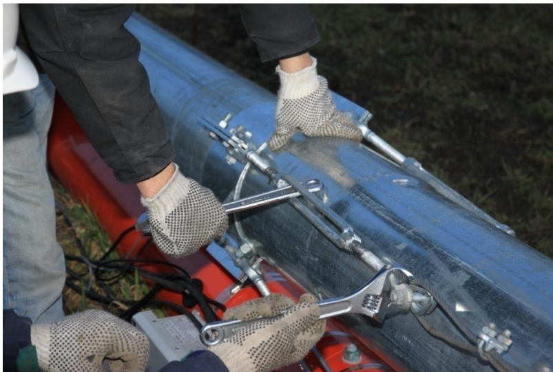
Picture 3-79: Tightening turnbuckles
