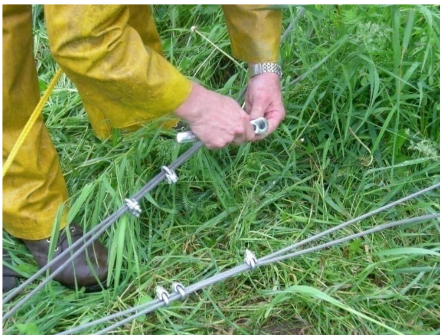
Picture 3-35: Wire rope clip guy wires together at anchor points
