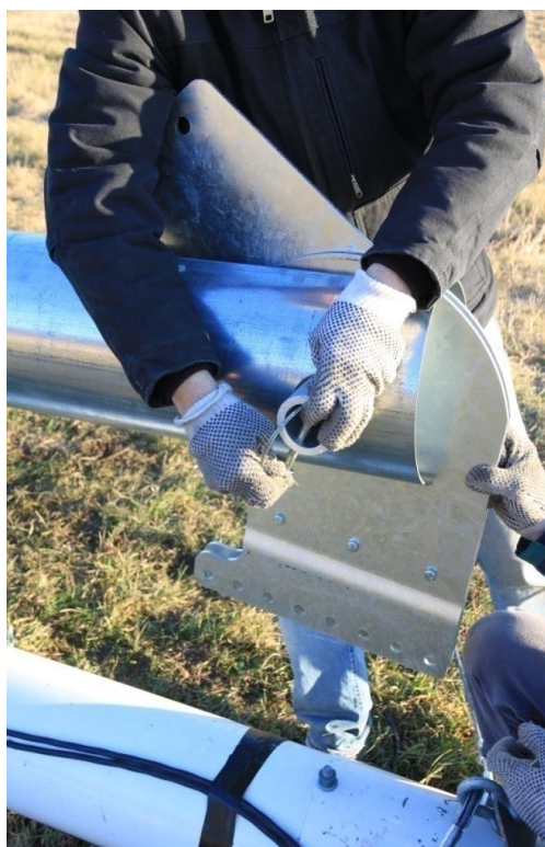
Picutre 3-55: Secure ginpole rocker plate pivot pipe
