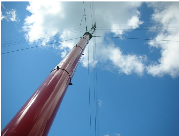
Picture 4-5: Straightening your tower
