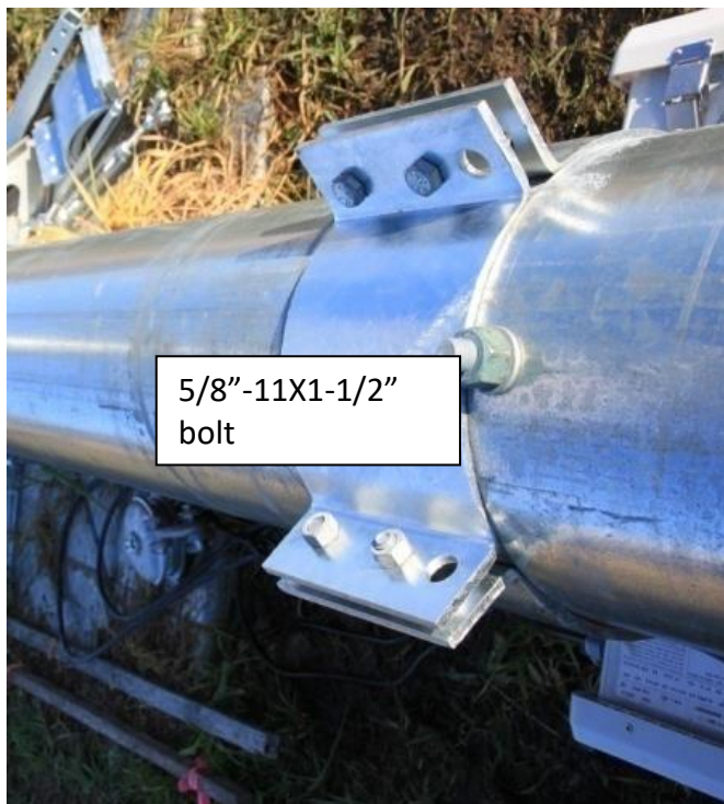
Picture 3-41: Ginpole jumper strut end-flange bolts
