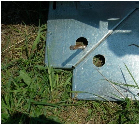
Picture 3-12: Ground Rod Placement
