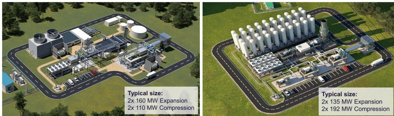
Figure 9 Schematic of Diabatic (left) and Adiabatic (right) CAES [21].
