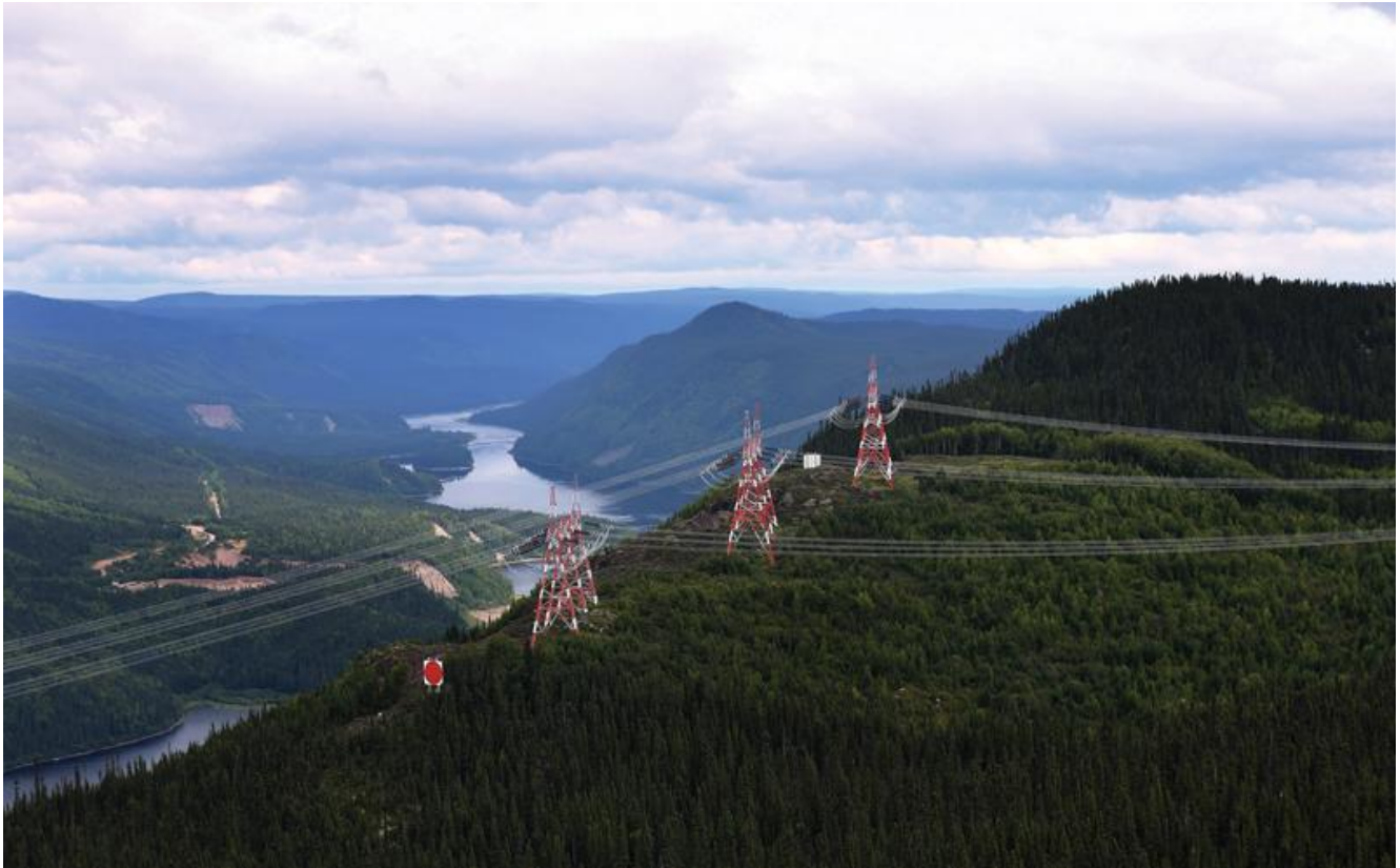
High-voltage transmission at the Churchill Falls hydroelectric power plant (Newfoundland and Labrador Hydro)
