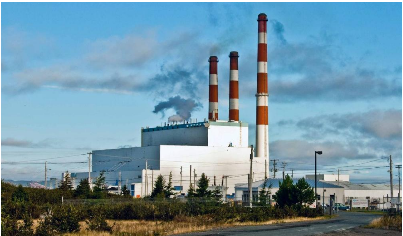
Holyrood Thermal Generating Station (Stantec)
