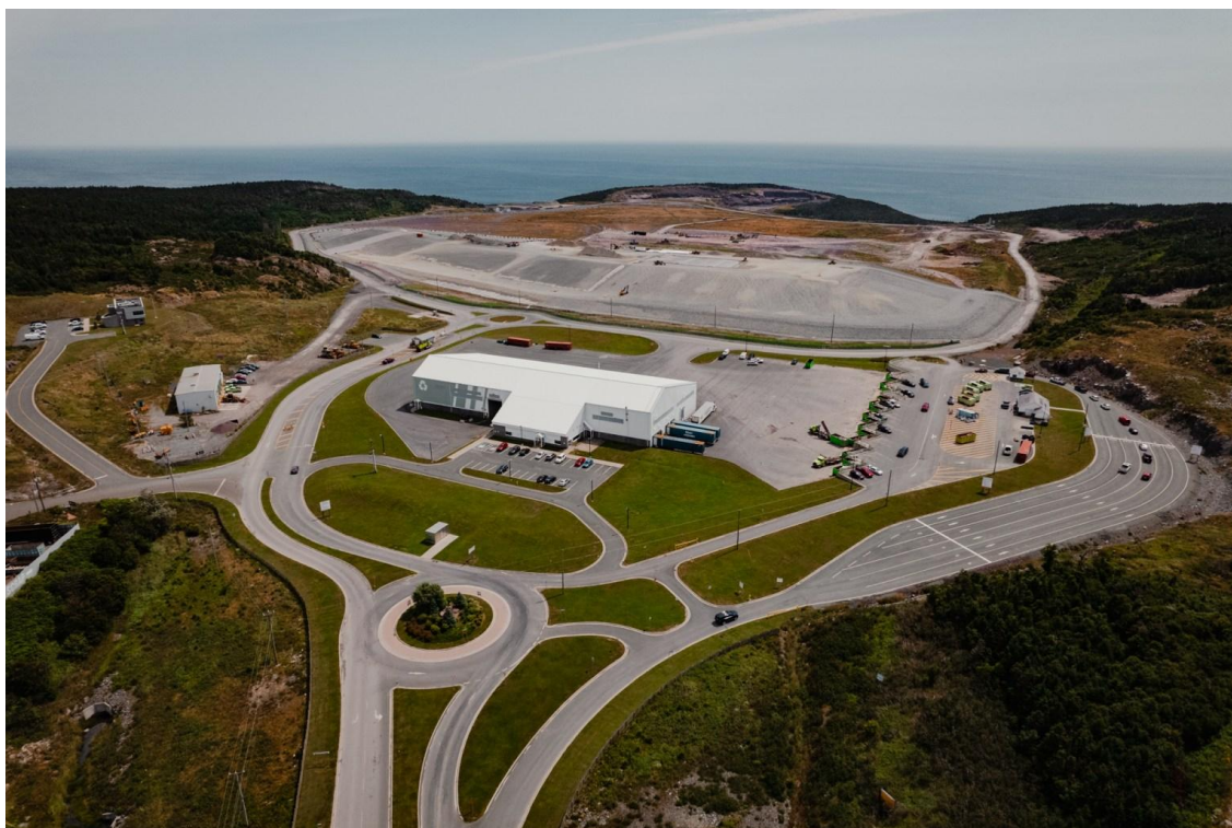
Robin Hood Bay Waste Management Facility in St. John's, NL (Tract Consulting Inc.)
